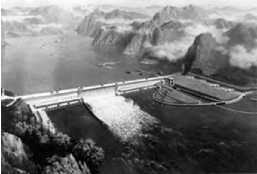
Figure 12.4 In this drawing of the completed Three Gorges Dam, the spillway to release water and control flooding is in the center, with electric generating plants on either side. On the right is a shiplift for comparatively small vessels, and on the far right is the five-step shiplock, which will allow ocean-going vessels to travel up the Yangtze to the western reaches of Chongqing.
